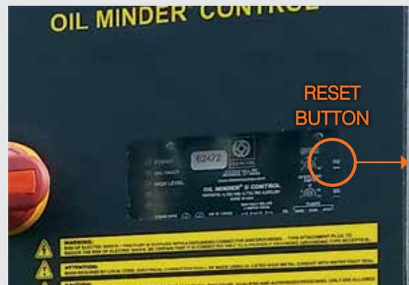
Push-to-test button ensures Oil Minder is properly installed and can be used to exercise the system.
