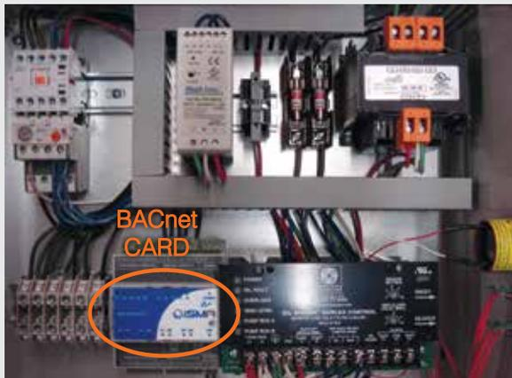
Oil Minder's integrated BACnet solution features a card in the control panel and can communicate with any protocol.
