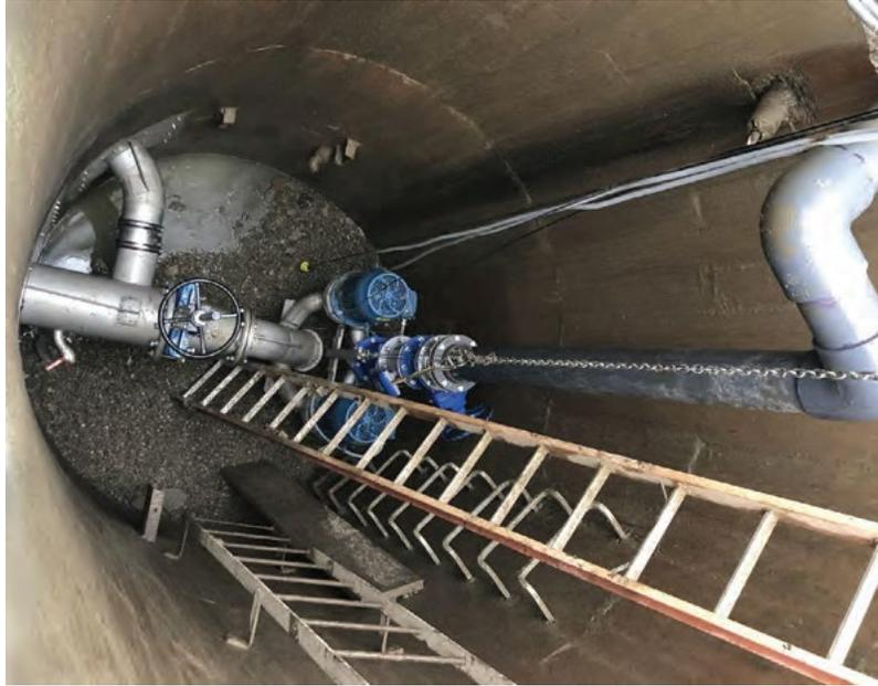
*Figure 4: The complete system installation shows a dry space with easily accessible equipment in place of a hazardous wet well environment (Picture provided by the Village of Sherman, Treatment Plant Operator, May 2018)*
