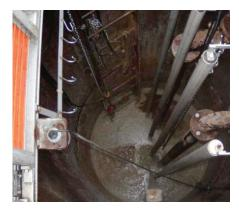
installed in a 20-foot-deep wet well, couldn't handle the plastic and failed often. Every time a pump clogged, a plant engineer had to raise the pump from the bottom of the sump and clean it out and repair it by hand—an effort that took about an hour of labor and put manufacturing operations at risk, as the wastewater system was running only on a backup pump.
