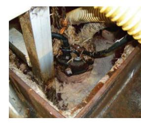
pellers that can shred almost anything they encounter and pass solids up to 31/2 inches in size. "There's enough torque in the SKs to keep them from plugging up," says Reid. "If they hit a bone, they just shear it." The SK55s have run nearly 12 hours a day since their installation with no unexpected failures, leading the company to use them for other applicationsandtodesignateBJM'sSKseriesas the plant's standard pump.
