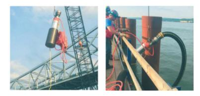
Stancor pumps were positioned to create a water supply line from the Hudson River to cure concrete properly on the bridge foundation. The construction process relied on a steady flow of water to maintain project timelines and structural integrity.
