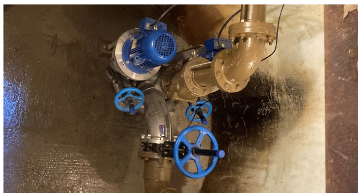
Figure 4: The complete system installation shows a dry space with easily accessible equipment in place of a hazardous wet well environment. (Picture provided by the Village of Sherman, as published in Treatment Plant Operator, May 2018 issue)
